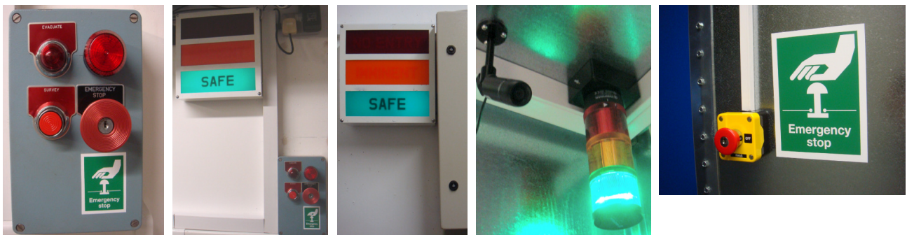
Figure 7: The room survey unit (left), the inner (SAFE – IMMINENT - RADIATION) and outer (SAFE – IMMINENT – NO ENTRY) status indicators (middle), one of the status indicators used in the Faraday cage (middle right) and of the 'panic' buttons (right).
